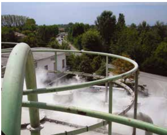
Silo workspace using spring-loaded valve
